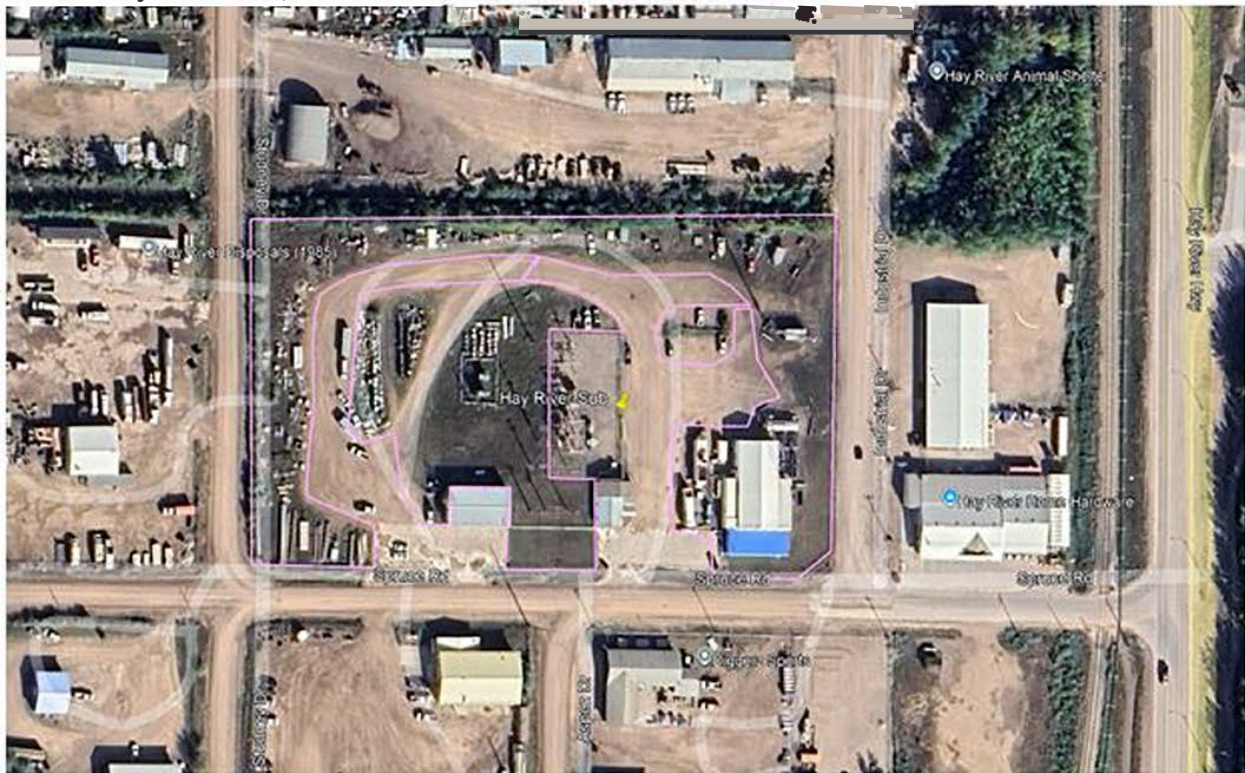
NTPC - Hay River Yard, Plant and Substation - 60.80642, -115.79748
