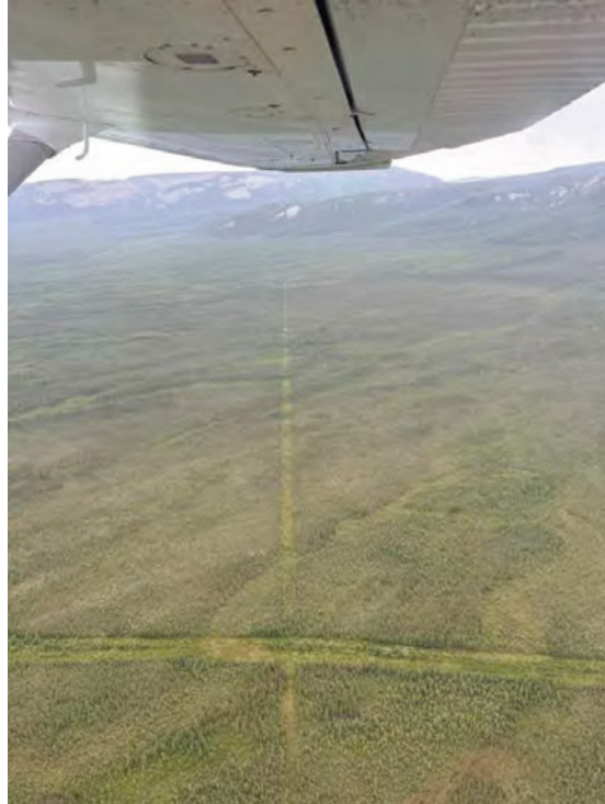
Photo 1: Pipeline/Road Alignment Vegetation
