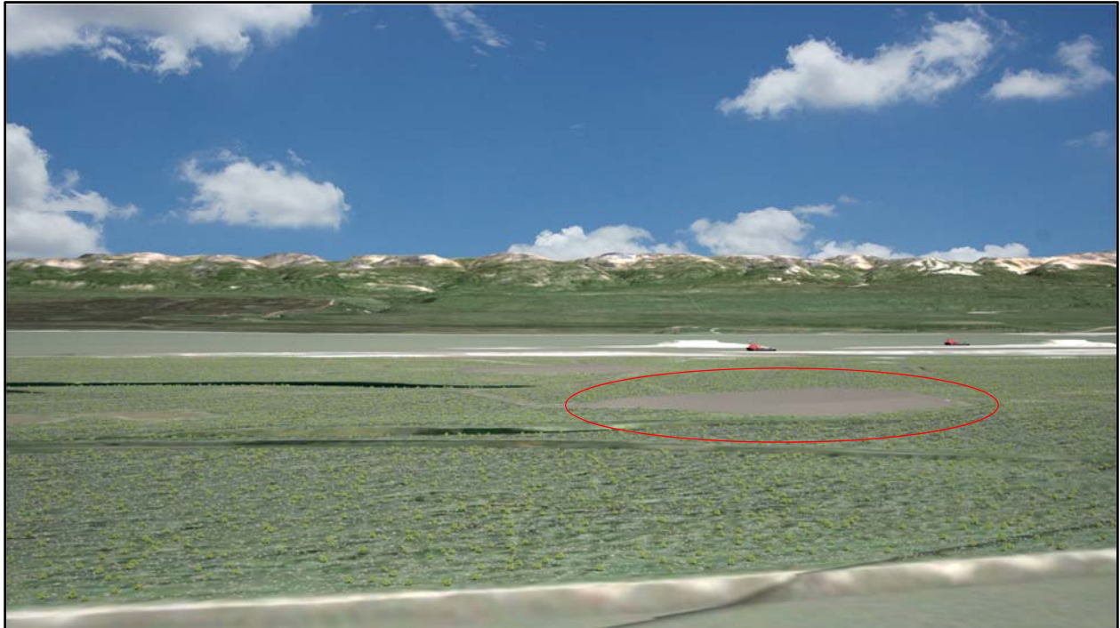
GIT view from River: Goose Island in the foreground with a view towards the Mackenzie River and the Norman Range on the horizon. The contoured former Goose Island Terminal pads are visible on the island (circled).
