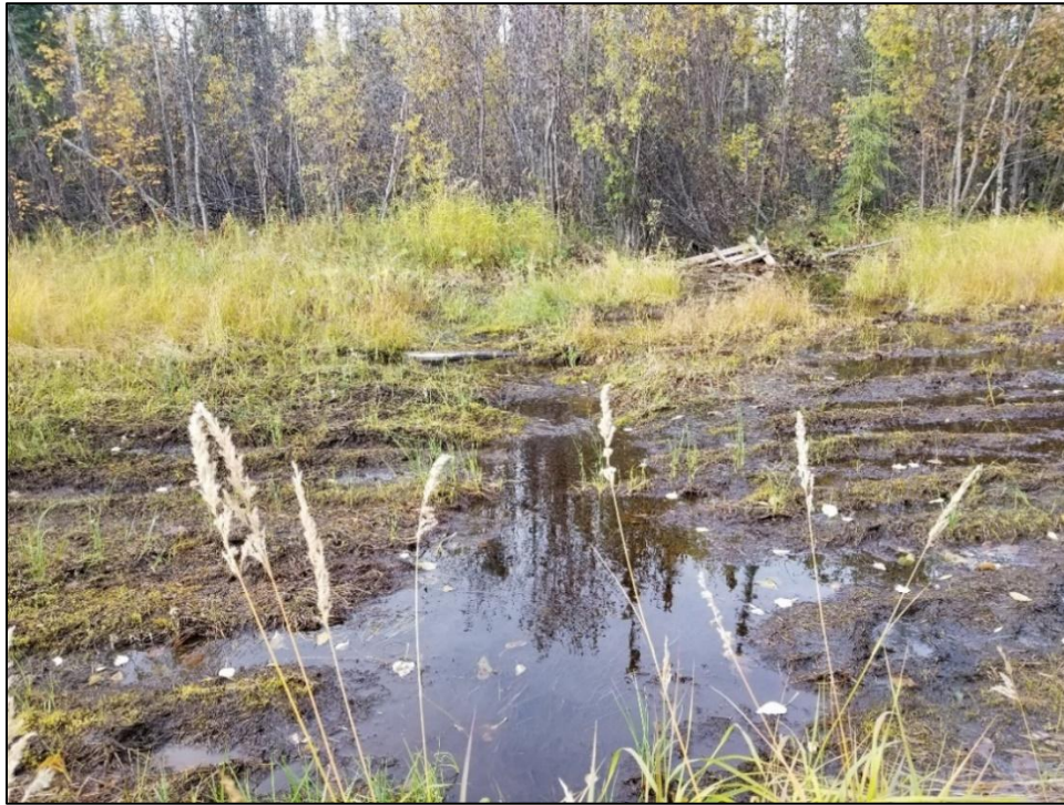
Photo 6: Drainage #4 looking west Approximately 1 L/s flowing to the east. No defined channels upstream or downstream of the alignment.
