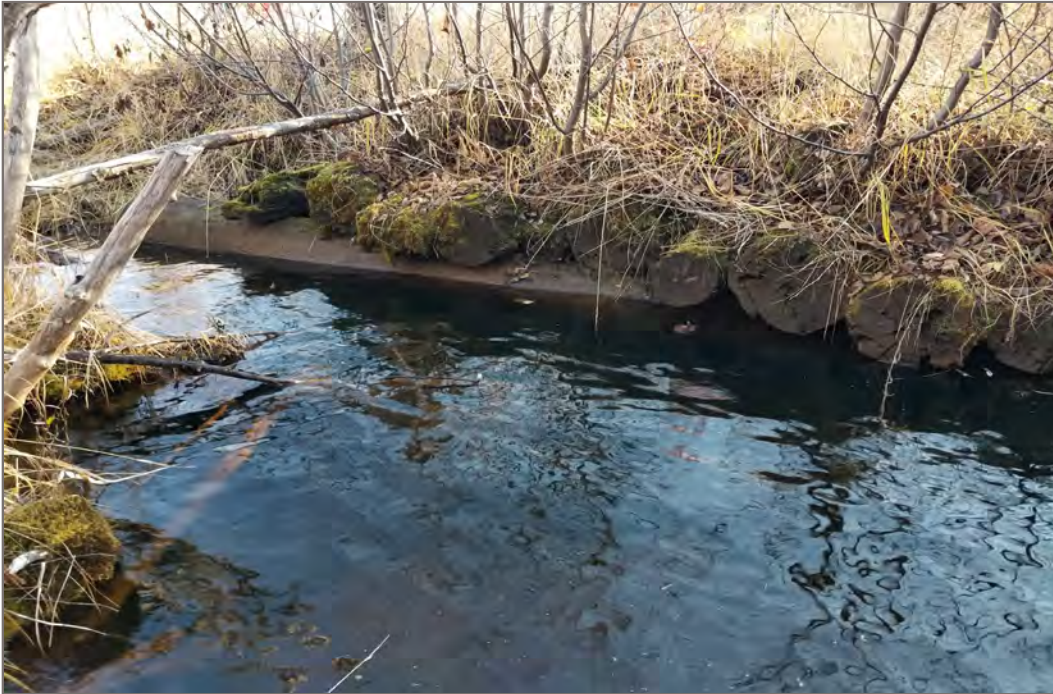
Photo 9: KM 812.7 (3 of 5) - Looking southeast (upstream) at downstream side of existing wooden bridge structure on winter road, downstream of proposed crossing.
