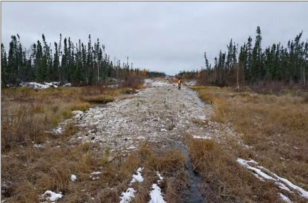
Photo 92: KM 919.9 (1 of 4) – Looking east along PDR alignment. A 600mm culvert backfilled with crushed rock span exists at this crossing.
