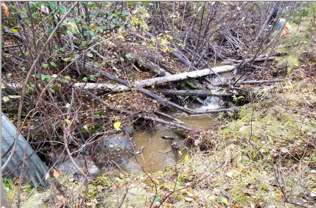
Photo 34: km 748.02 (6 of 7) – Looking upstream (northeast) from culvert inlet. Channel well defined with woody debris present.
