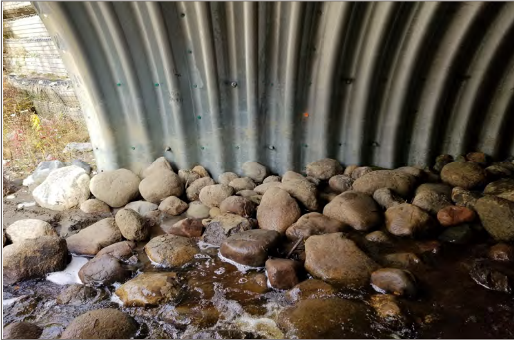
Photo 25: km 752.61 (4 of 7) – Looking at north wall at culvert outlet. Culvert in good condition. Mud lines indicate water has reached 0.65m outlet depth.
