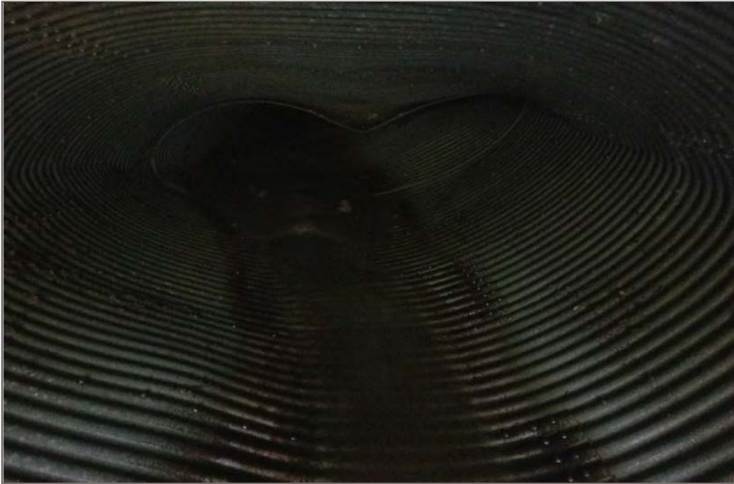
Photo 33: km 748.02 (5 of 7) – Looking downstream from inlet of culvert. Culvert severely damaged.
