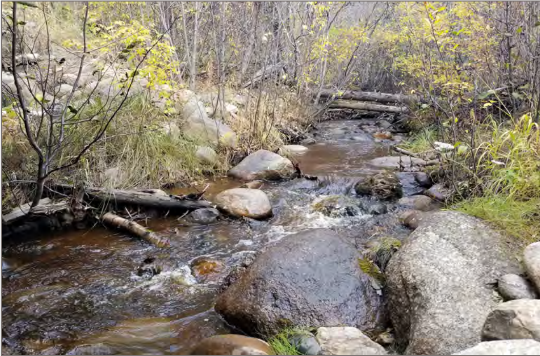
Photo 27: km 752.61 (6 of 7) – Looking upstream (east) at channel approaching existing culvert. Water confined within a well-defined and stable channel.
