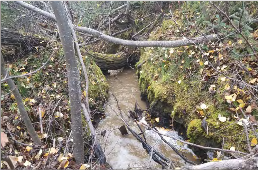
Photo 50: km 741.74 (3 of 3) – Looking east (upstream) approximately 40 metres downstream of the highway alignment.
