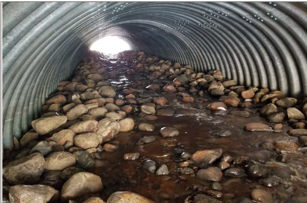
Photo 24: km 752.61 (3 of 7) – Looking upstream within culvert. Boulders throughout culvert with low flow channel centred within culvert.
