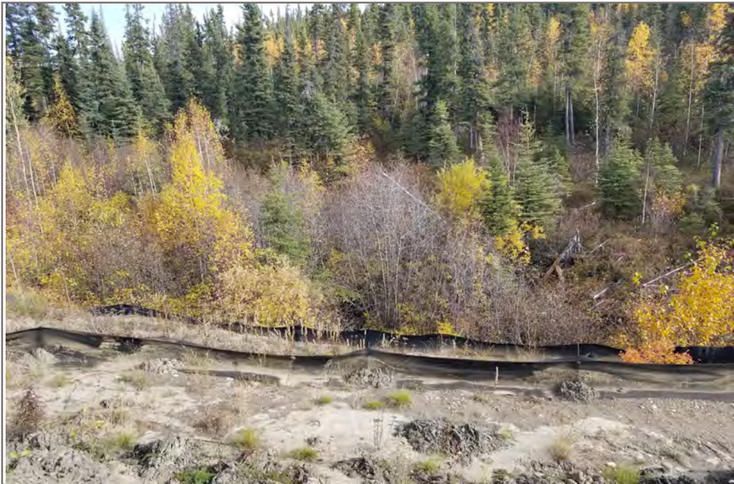
Photo 22: km 752.61 (1 of 7) – Looking upstream (east) from winter road alignment. MSE walls installed as headwalls for existing culvert.
