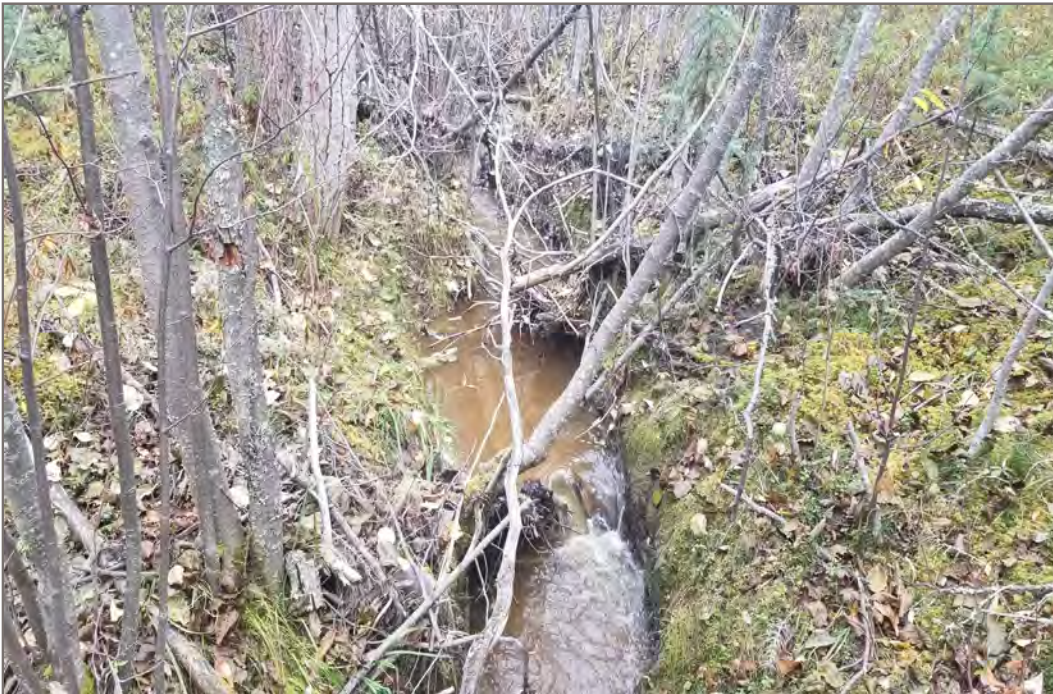
Photo 48: km 741.74 (1 of 3) – Looking east (upstream) approximately 75 metres upstream of the highway alignment. Woody debris present in a small channel.
