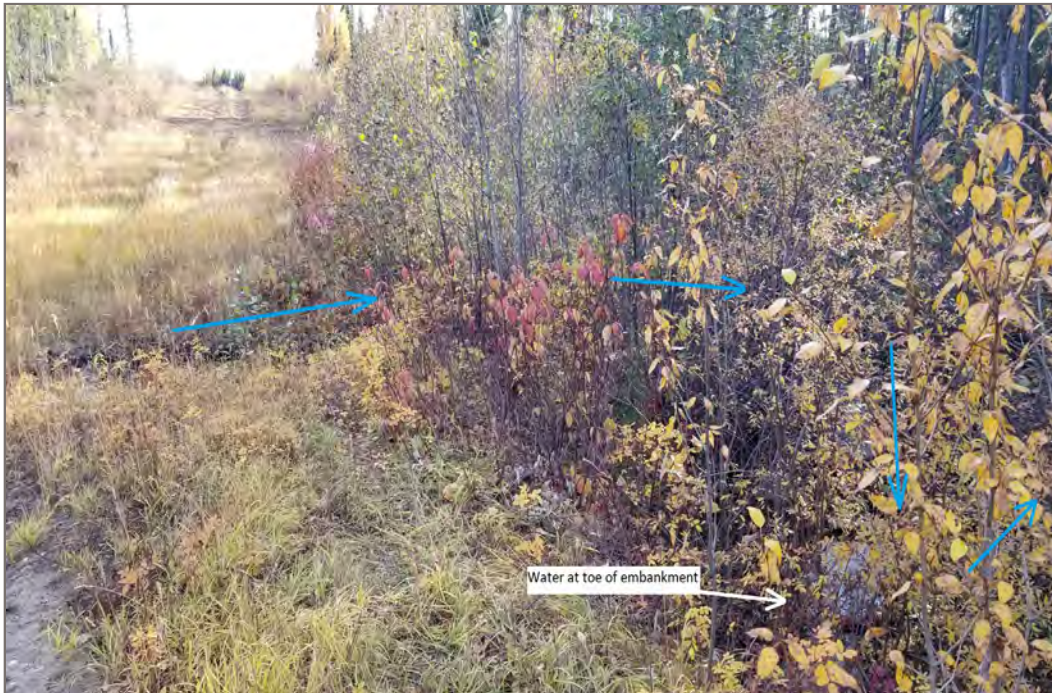
Photo 55: km 739.55 (3 of 4) – Looking south along highway alignment. Blue arrows indicate flow path. Downstream of the alignment the channel takes a 135 degree turn north, coming back to the toe of the existing roadway.
