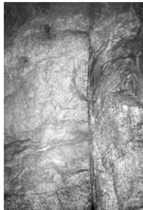
Figure 5: In-situ open fracture
