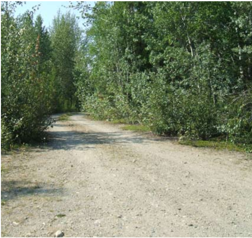
FIG 2.9 Minimizing per hectare costs can be an important objective on long, linear projects; for instance when decommissioning trails or temporary roads. The same principles of good ground preparation and implementation apply, but they need not be complicated. Decompacting this roadbed with a ripper or large disk, followed by fertilizing and seeding with a basic seed mix (3 – 4 appropriate species) will suffice. The vast majority of work and expense on these projects occurs where the road or trail intersects a slope or water body. In those locations, more extensive erosion control measures are required.
