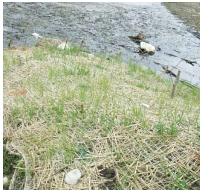
FIG 3.12c Grass and willow cuttings growing through the blanket the following spring.
