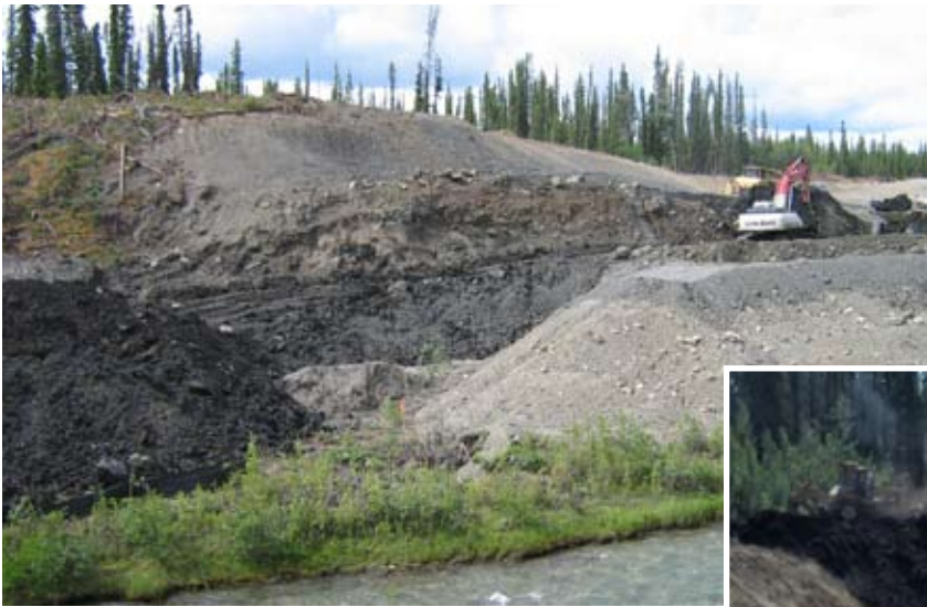
FIG 3.7 Saving organics. Surface organic material is being hauled and stockpiled at this site for reapplication after construction is completed. This effort, which required planning ahead and good communication between the site manager and contractor, will pay huge dividends in the revegetation results and significantly reduce fertilizer and seed cost.
