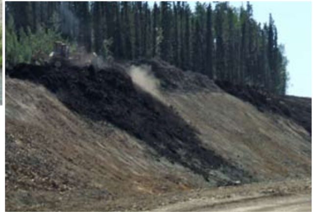
FIG 3.7 Saving organics. Surface organic material is being hauled and stockpiled at this site for reapplication after construction is completed. This effort, which required planning ahead and good communication between the site manager and contractor, will pay huge dividends in the revegetation results and significantly reduce fertilizer and seed cost.
