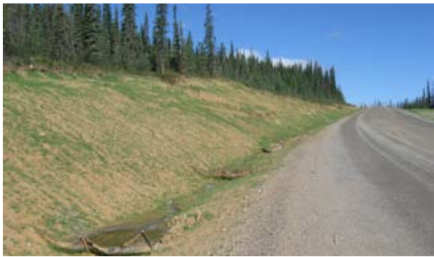
(i) Instead of track-walking and conventional seeding, this slope was hydroseeded (same slope depicted in photo d). Note how seeding was correctly extended all the way to the edge of the roadbed ( i.e. , seeded on both sides of the ditch). This will help stabilize the roadbed and prevent the spread of invasive plants. Also note the installation of temporary check dams in the ditch to slow the velocity of flowing water until vegetation is established.
