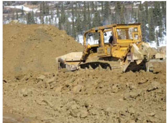
FIG 3.8 Ground should be decompacted before organic materials are spread.
