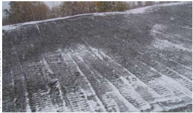
(f) This slope has been properly trackwalked. Notice how the tractor was driven up-slope, rather than cross-slope. The result is that cleat tracks run perpendicular to the slope and serve as catchments for seed, fertilizer and surface water.
