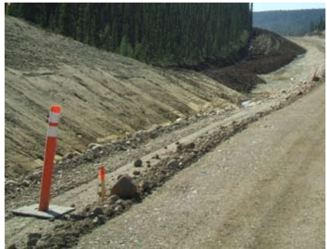
Fig 5.6 All types of site conditions can be encountered when revegetating highway right-of-ways, calling for the application of many different tools in the planners toolbox. Revegetating right-of-ways also requires advanced planning and logistics, because the work must be coordinated with road designers and contractors. The main objectives are to protect the roadbed, reduce road hazards, enhance visual aesthetics, reduce future maintenance costs, and exclude woody and invasive species.
