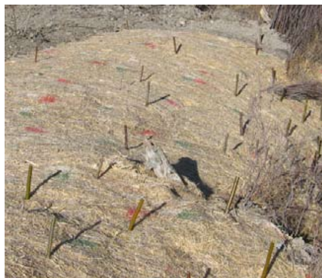
FIG 4.28 Vertical willow-staking through a jute-straw erosion control blanket
