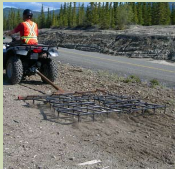
FIG 4.17 Seed being covered using the small tine harrow pictured in Fig. 4.15. Note the limited penetration of the tines on this gravelly surface. In this case, the ground was harrowed twice to increase the amount of seed-soil contact.
