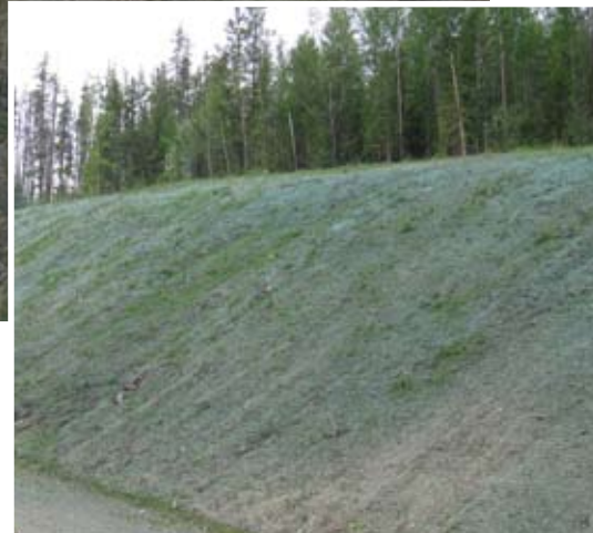
FIG 5.3 Hydroseeding can be a good option on steep slopes.
