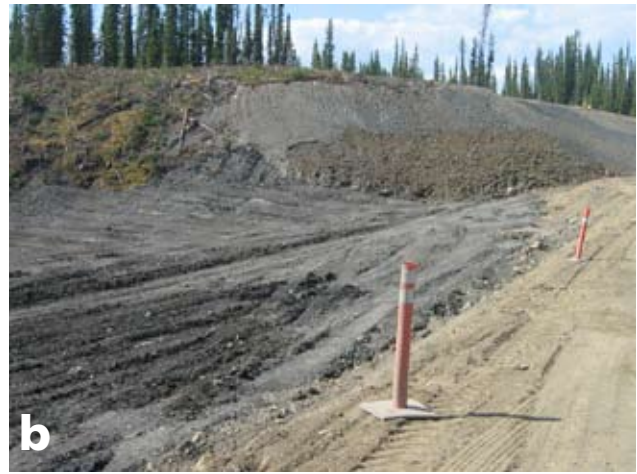
b: Same site as photo a after soil and organics were placed over the melting permafrost. This provided insulation and halted the melting process.
