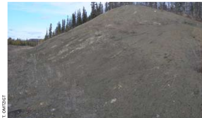
FIG 3.9 Preparing the surface of steep slopes.
