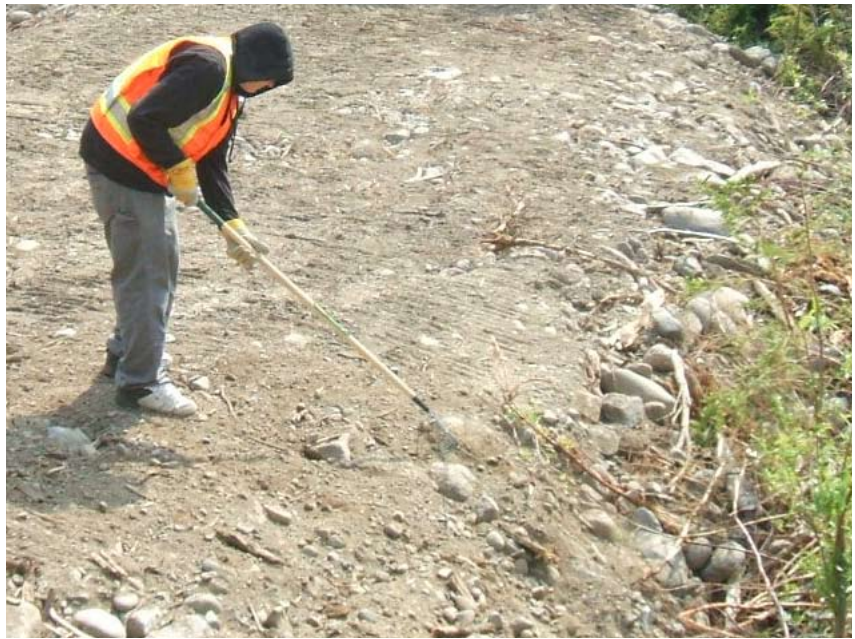
FIG 4.23 Nearly all sites will require some hand-work to cover seed and fertilizer in places where equipment cannot operate.
