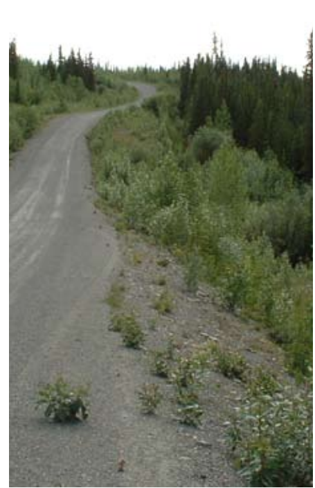
FIG 2.10 This Yukon roadside has been left to revegetate naturally, with no seeding. Soon, the woody species growing up to the roadbed will impede driver visibility and will need to be cleared. If the site had been seeded with grasses, the growth of woody species could have been impeded, resulting in reduced maintenance costs.
