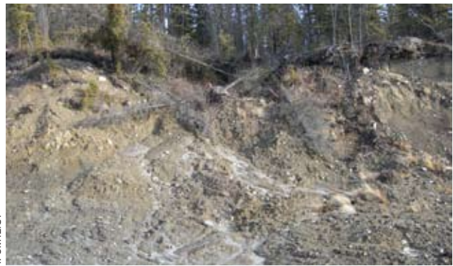
(j) Revegetation cannot be used to solve every slope issue, at least not alone. This slope is slumping for two reasons. First, the slope was cut at a steep angle into unconsolidated fill (glacial till) that is difficult to stabilize. Second, the situation is aggravated by the presence of a small drainage that runs off onto the newly exposed surface. Solution: control (divert or channel) drainage, decrease the slope angle and consider bioengineering solutions (see Chapter 4). Only then will the surface be stable enough for seeding.
