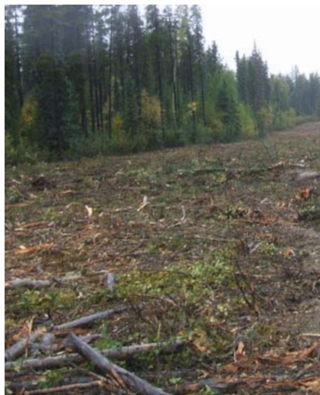
FIG 2.14. Sites that are only cleared or grubbed, and where the organic soil layer is left intact, usually will revegetate quickly on their own – with results that are as good as or better than seeding. Even if the organic layer was disturbed, a light seeding may be all that is required if enough organics soil remains in place and there is low risk for erosion.
