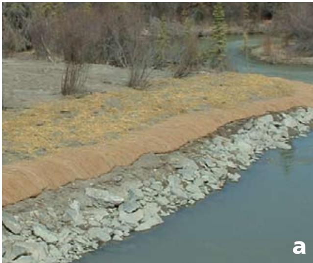
FIG 4.30 A three-pronged approach to bank revegetation. A willow hedge was constructed closest to the water's edge using stakes and an erosion control blanket (closeup in b), followed by mulch and seeding above. The willow bushes above the mulch were translocated from a donor site just a short distance away.
