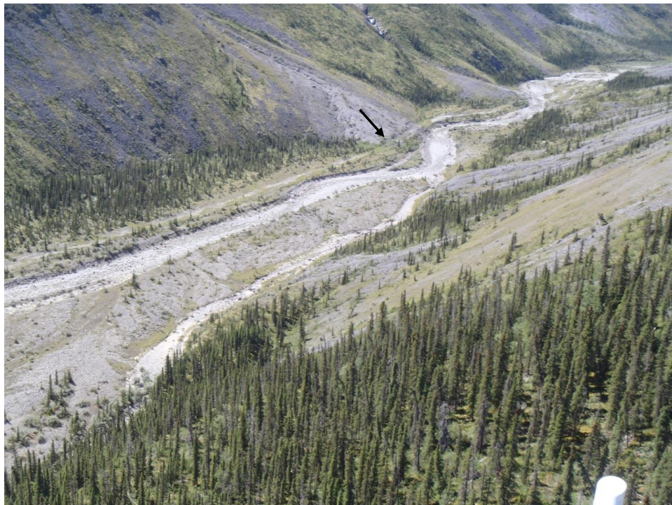
Figure 8 Sundog Creek at Km 31.7 – oblique air-photo showing location of proposed road, using historical right of way.
