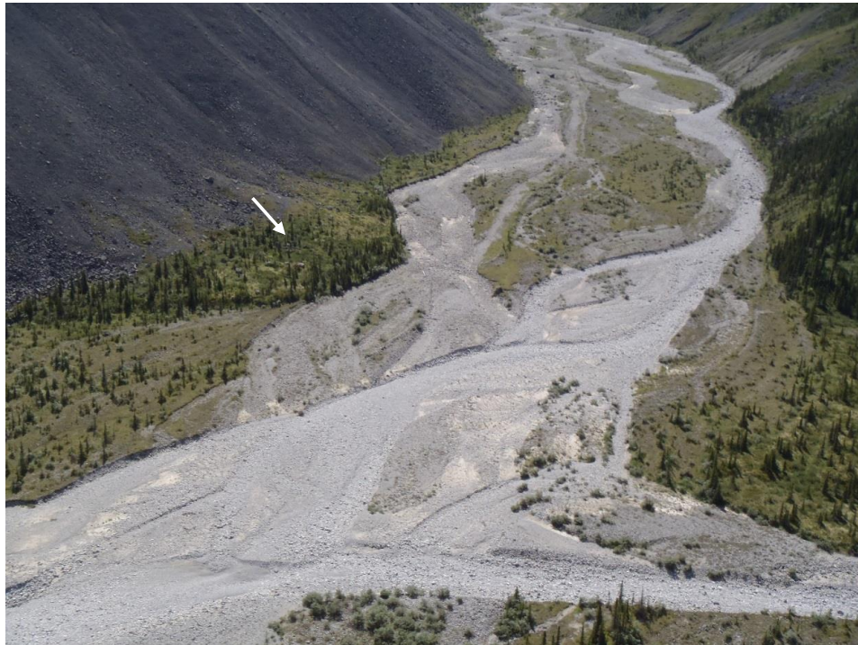
Figure 10 Sundog Creek at Km 34.7 – oblique air-photo showing location of proposed road.
