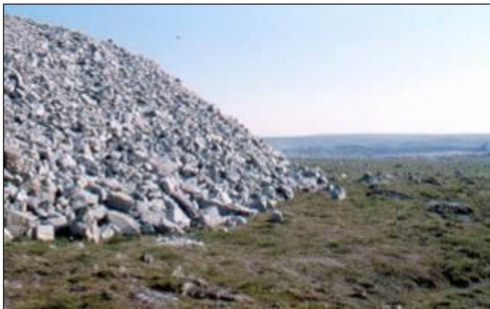
Plate 2.4-2. Typical WRSA embankment (note large fragmentation that encourages cool air flow).
