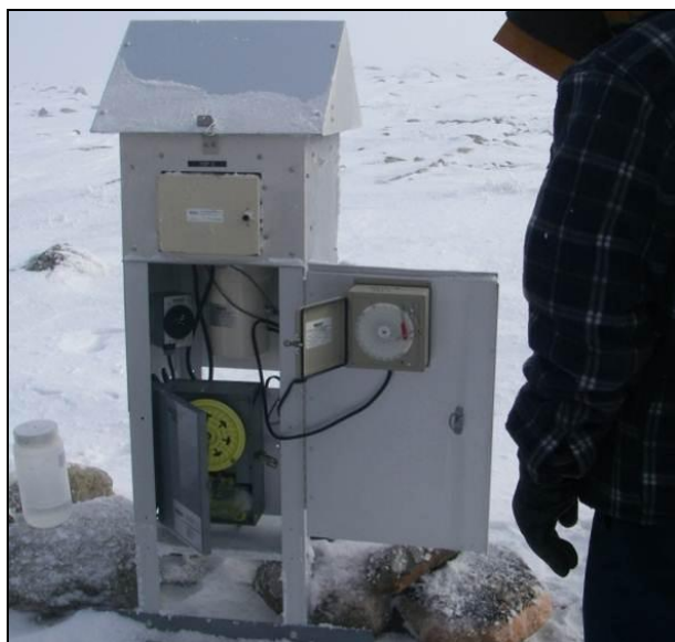
Plate 5.1-1. HVAS station TSP-3, exposed interior view, May 2011.
