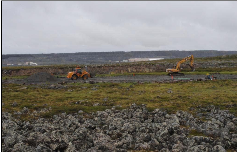
Plate 7.4-1. Erosion control construction work near the Panda Diversion Channel, August 2011.
