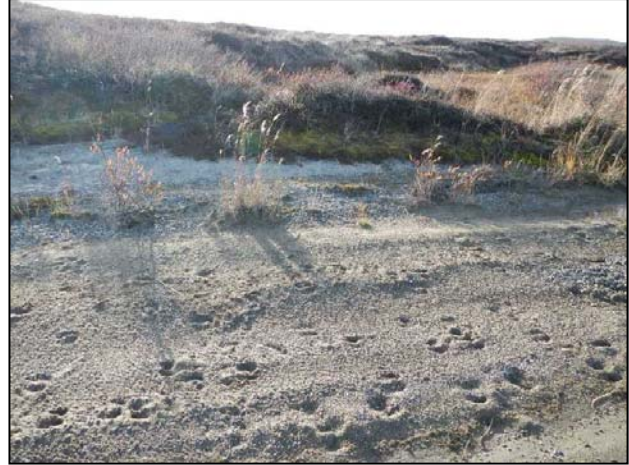
Photo E5-SL57: Sandy shoreline detail with steep banks and some bank failures (looking west)
