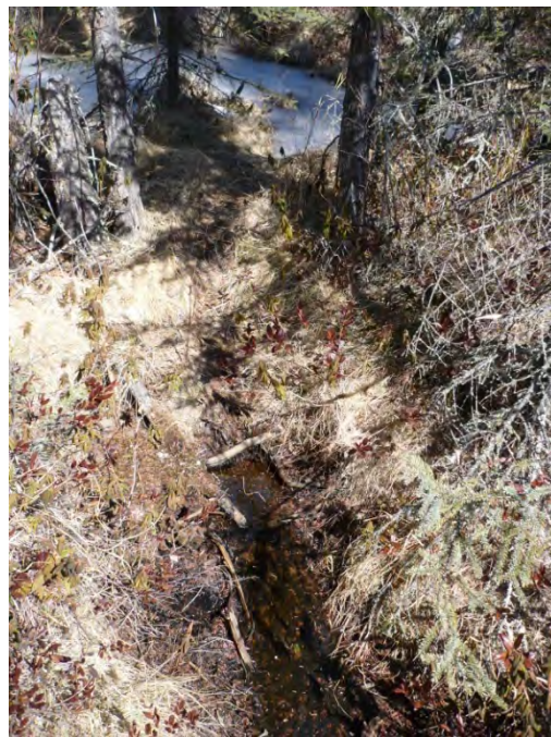
Photo 10: South Tardiff Out looking upstream at an earth dam, May 2009
