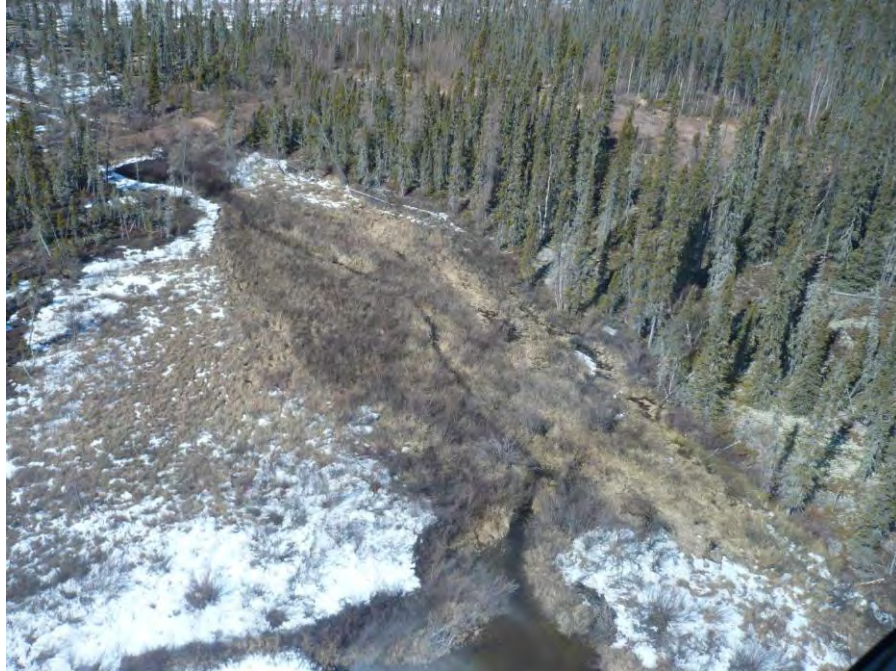
Photo 1: Aerial view of Fred Out, showing outlet from Fred and culvert under road. May 2009.
