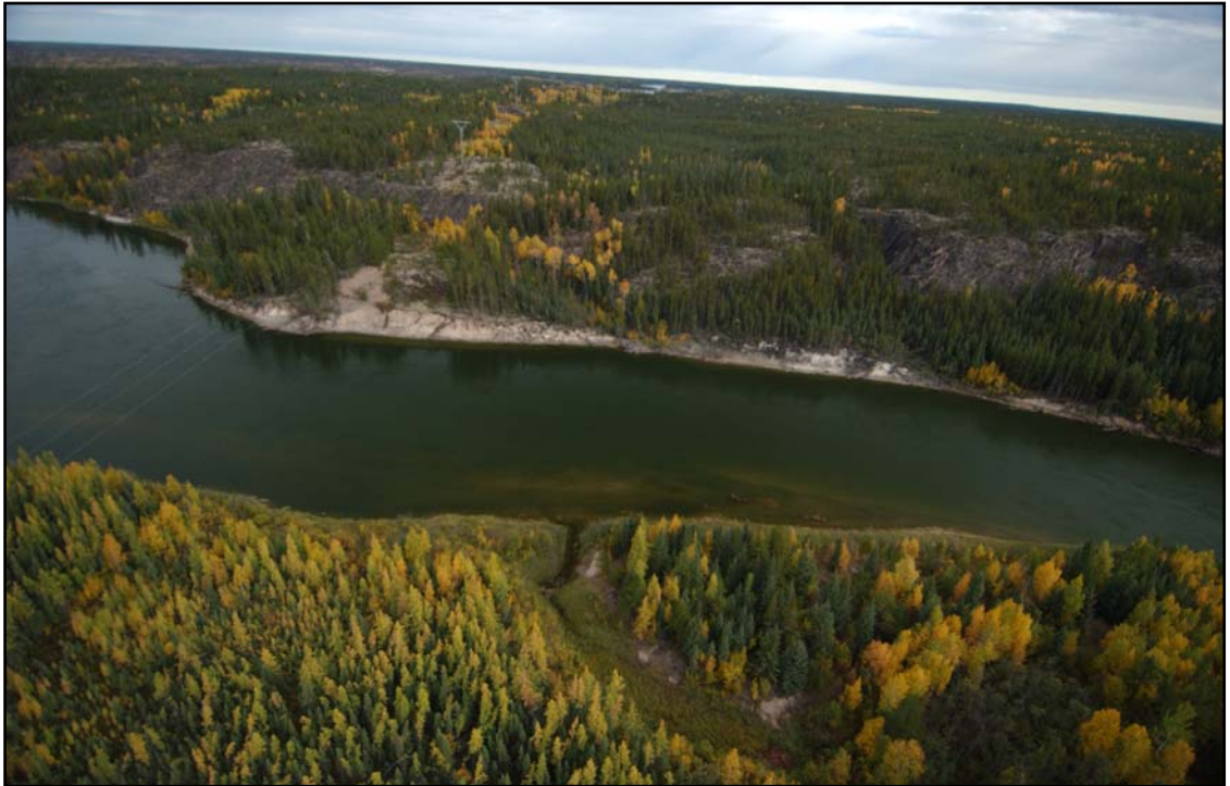
Plate 8-10: Existing Twin Gorges Transmission Line – Example of River Crossing
