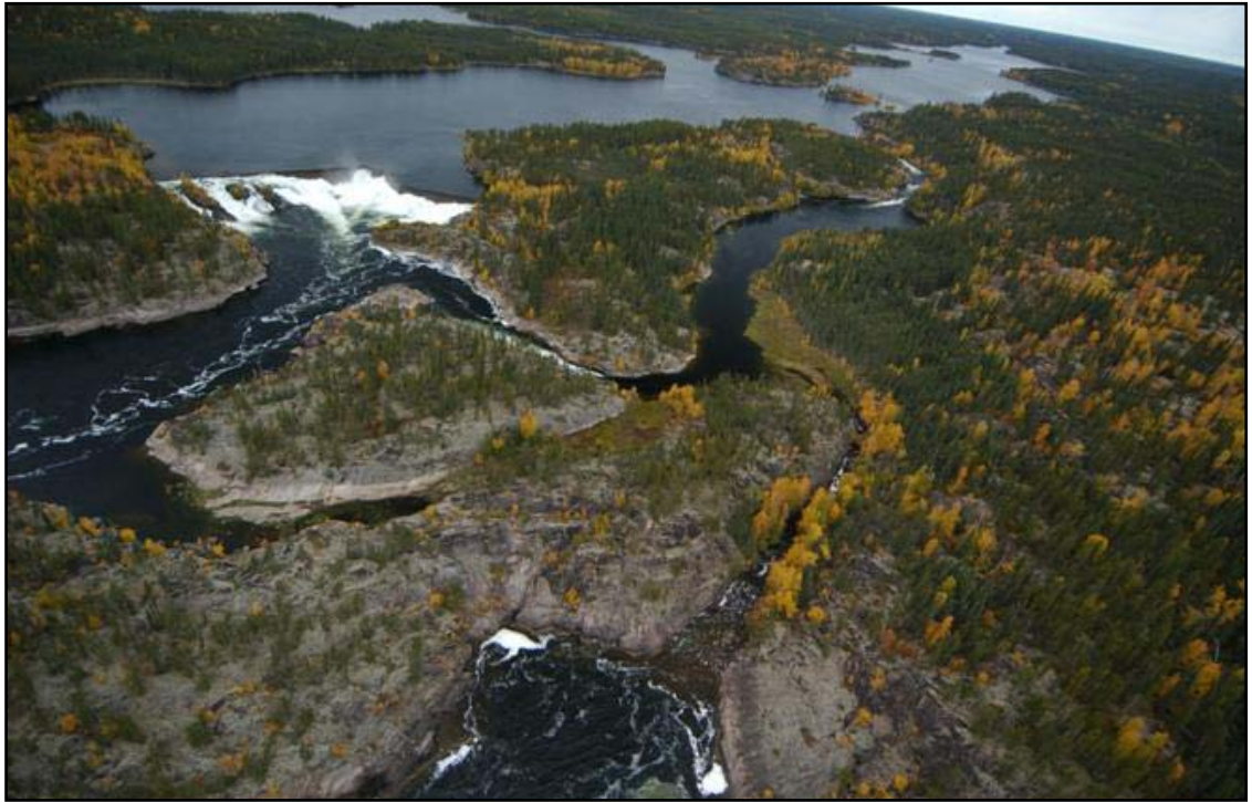
Plate 8-4: South Valley Spillway looking upstream at the Taltson River
