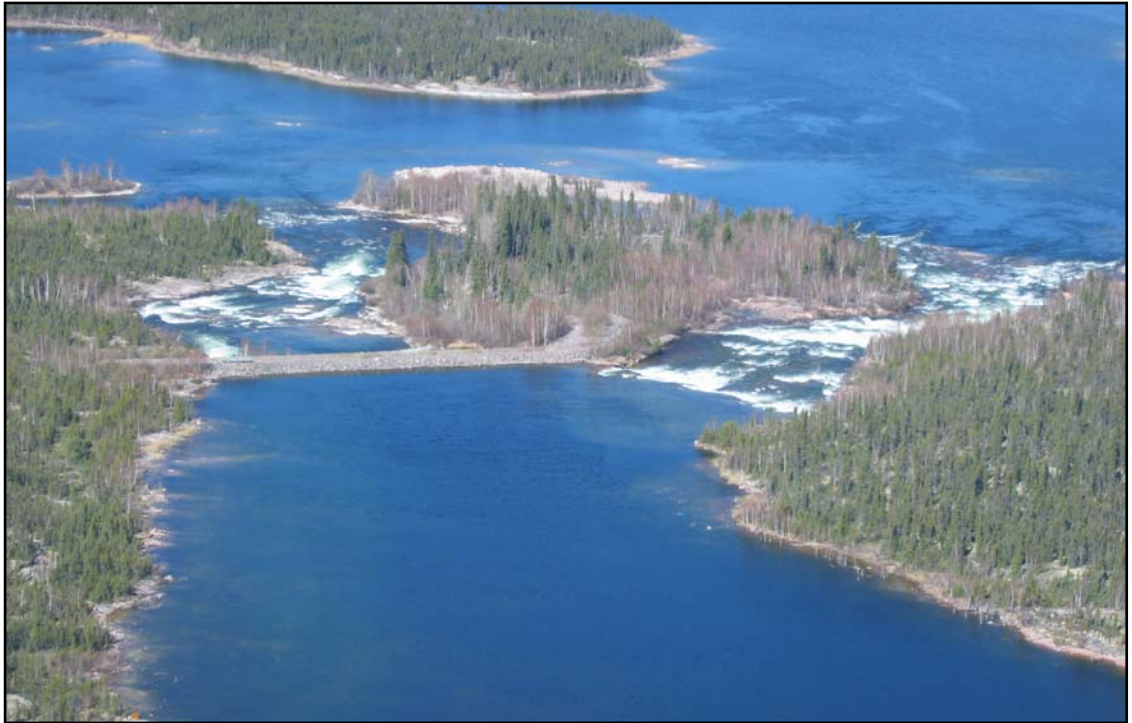
Plate 8-8: Nonacho Lake Control Structure
