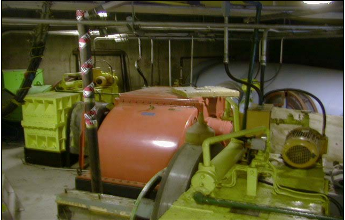
Plate 8-12: Ossberger Turbines
