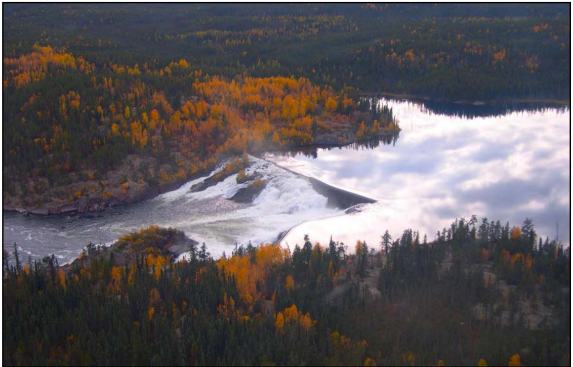
Plate 8-5: South Valley Spillway
