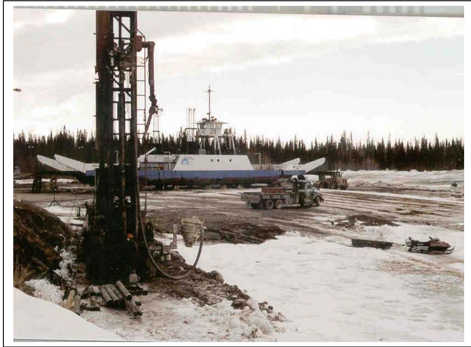
Photo 3: April 18, 2003 – Drilling at A-1, looking south to Merv Hardie Ferry
