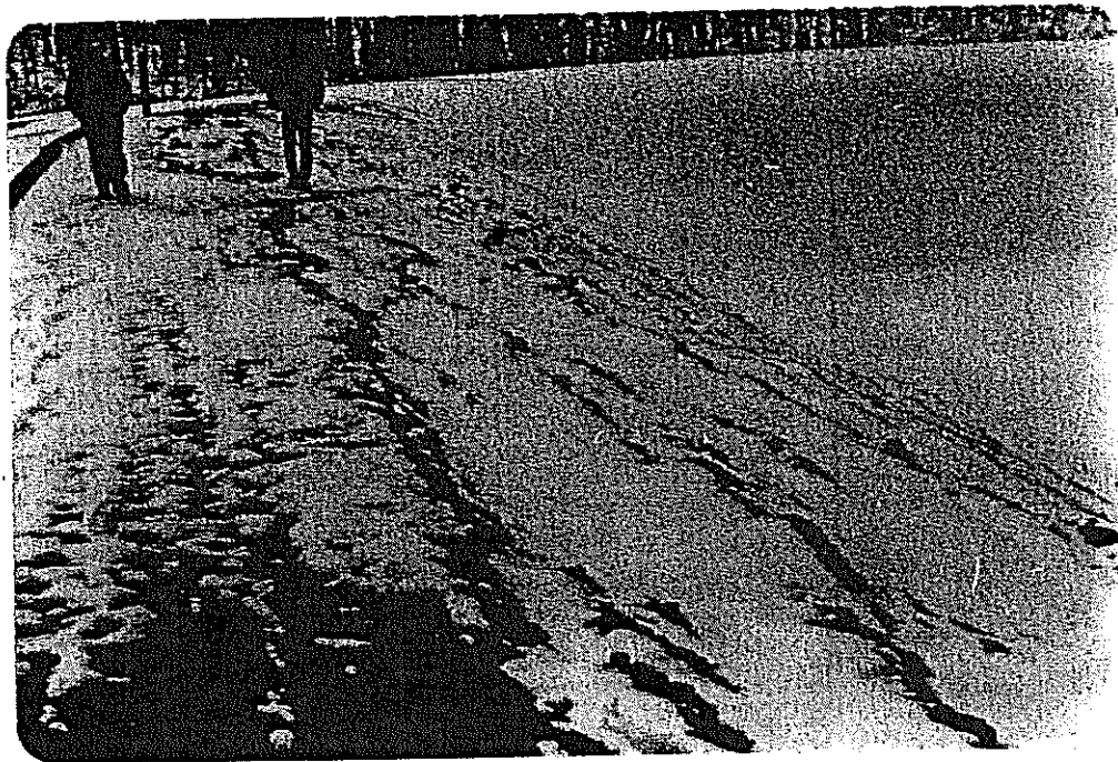
Photo 9: Movement of Gravel Protection Blanket.
