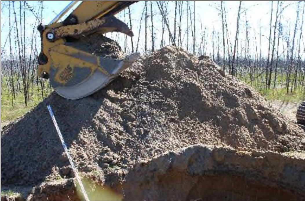
Photo 15: Prospect 13C-06. Spoil pile of fine grained sand. Photo taken July 12, 2017
